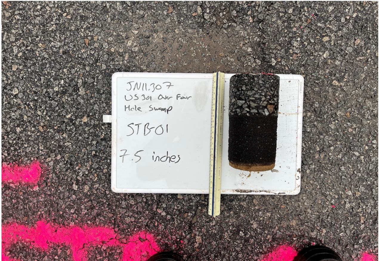
Photograph 1: Asphalt Core STB-01
