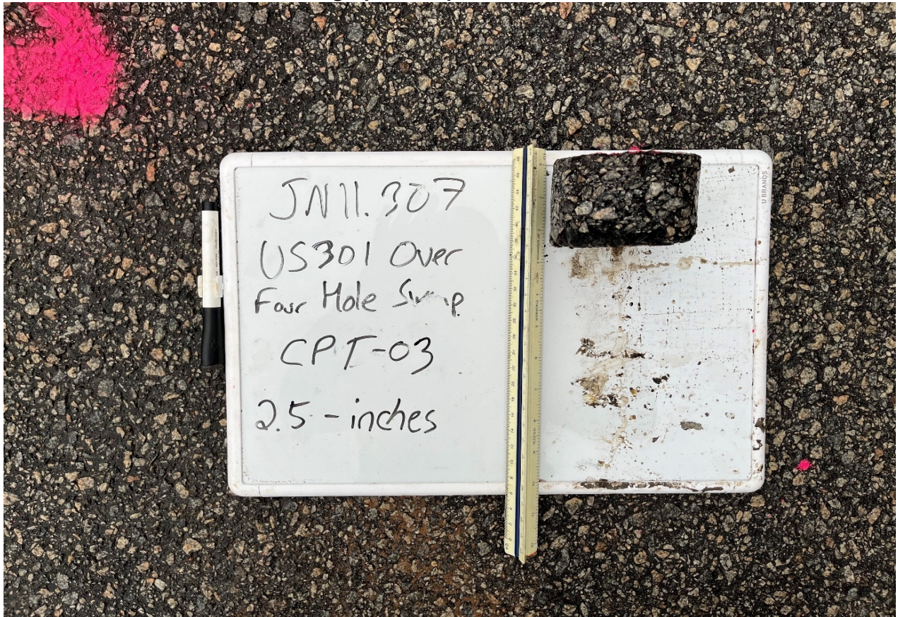
Photograph 7: Asphalt Core CPT-03
