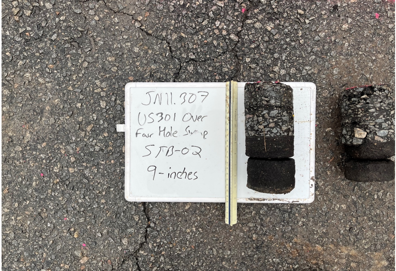
Photograph 2: Asphalt Core STB-02
