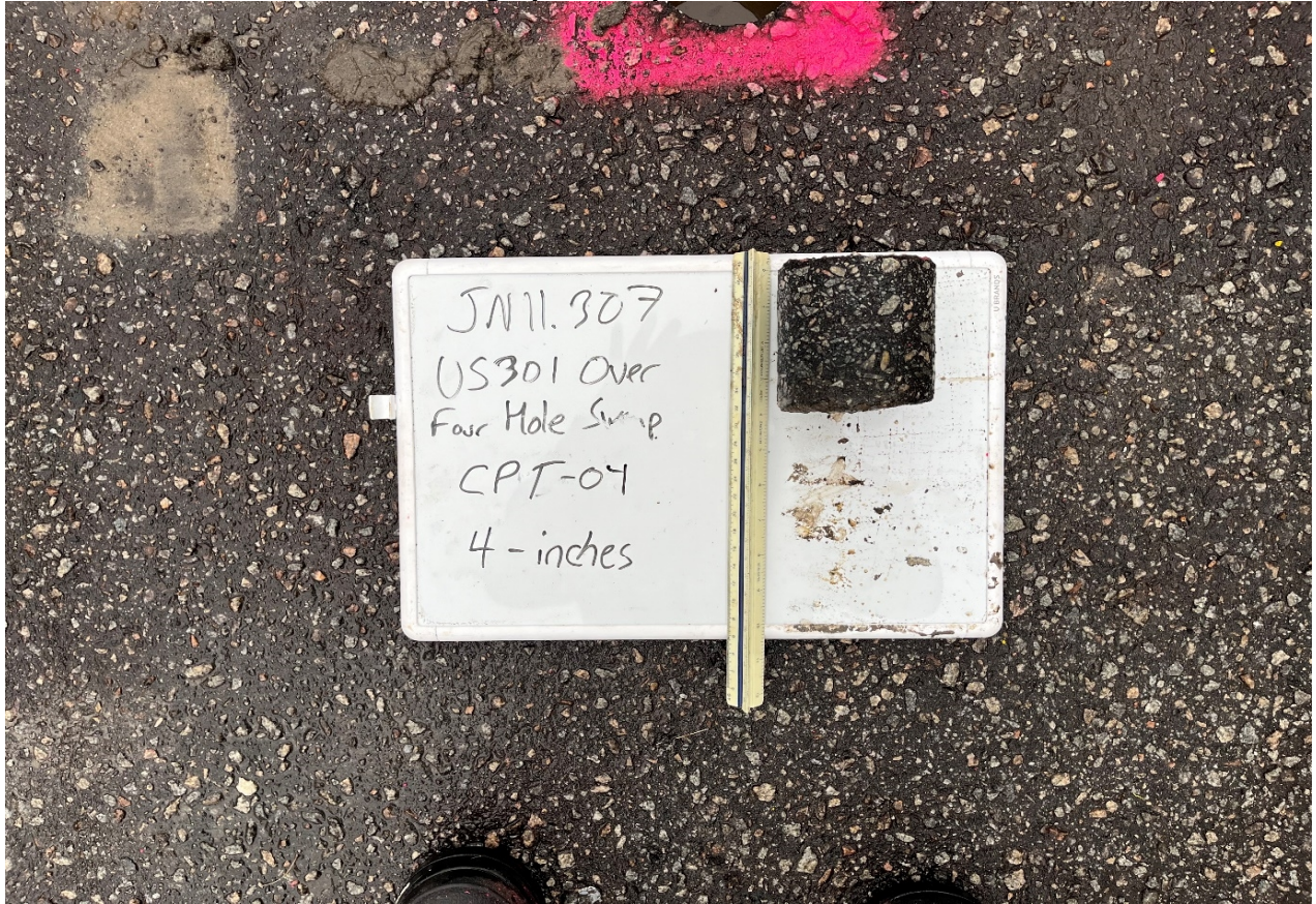
Photograph 8: Asphalt Core CPT-04
